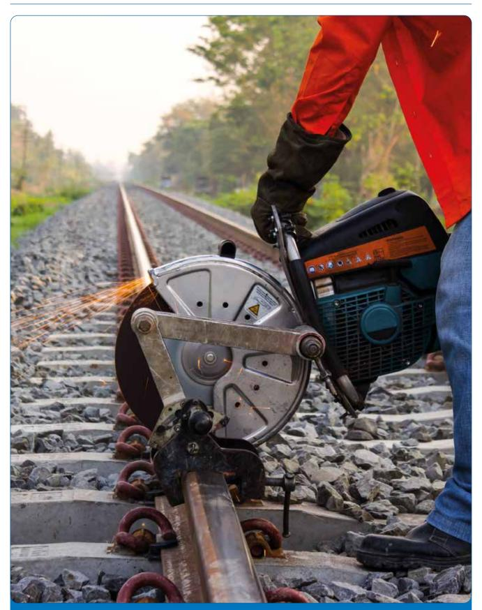
Karbosan high performance Rail Cut-Off Discs, cut all rails in different hardness and weights, quickly and without vibration. Because of the high number of cuttings made with a single Disc, the worker avoids waste of time by not changing the disc constantly. The Rail Cut-Off Disc provides a smooth structure on the rail surface. Zirconium and Aluminum Oxide abrasive products are suitable for all kinds of rails.
